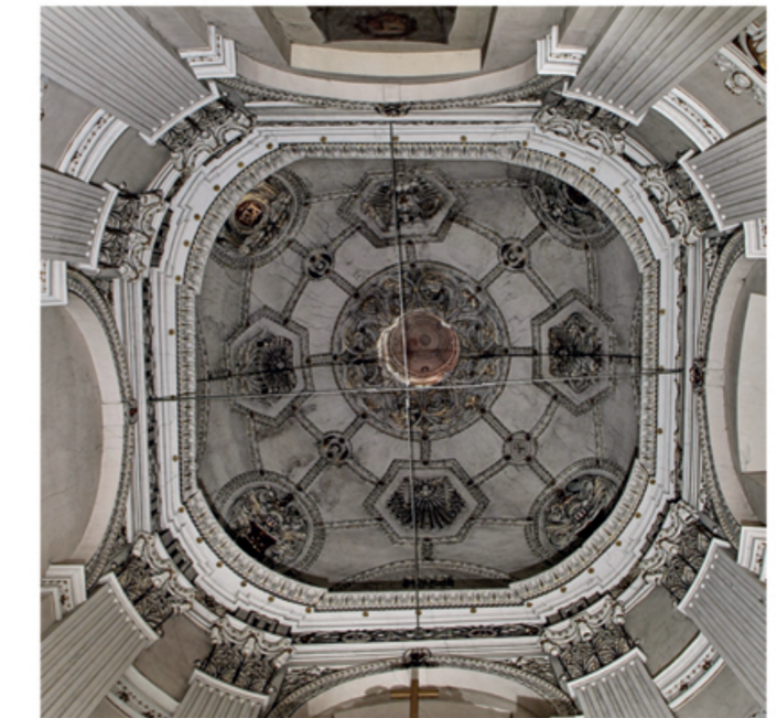
Vault in Firlej's chapel
